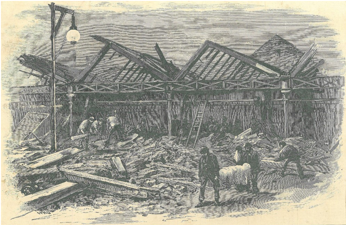
THE WEAIVING-SHED, WHERE THE BODIES OF THOSE KILLED WERE "FOUND." FALL OF MESSRS. J. AND J. TEMPLETON'S CARPET FACTORY, GREENHEAD, GLASGOW.
