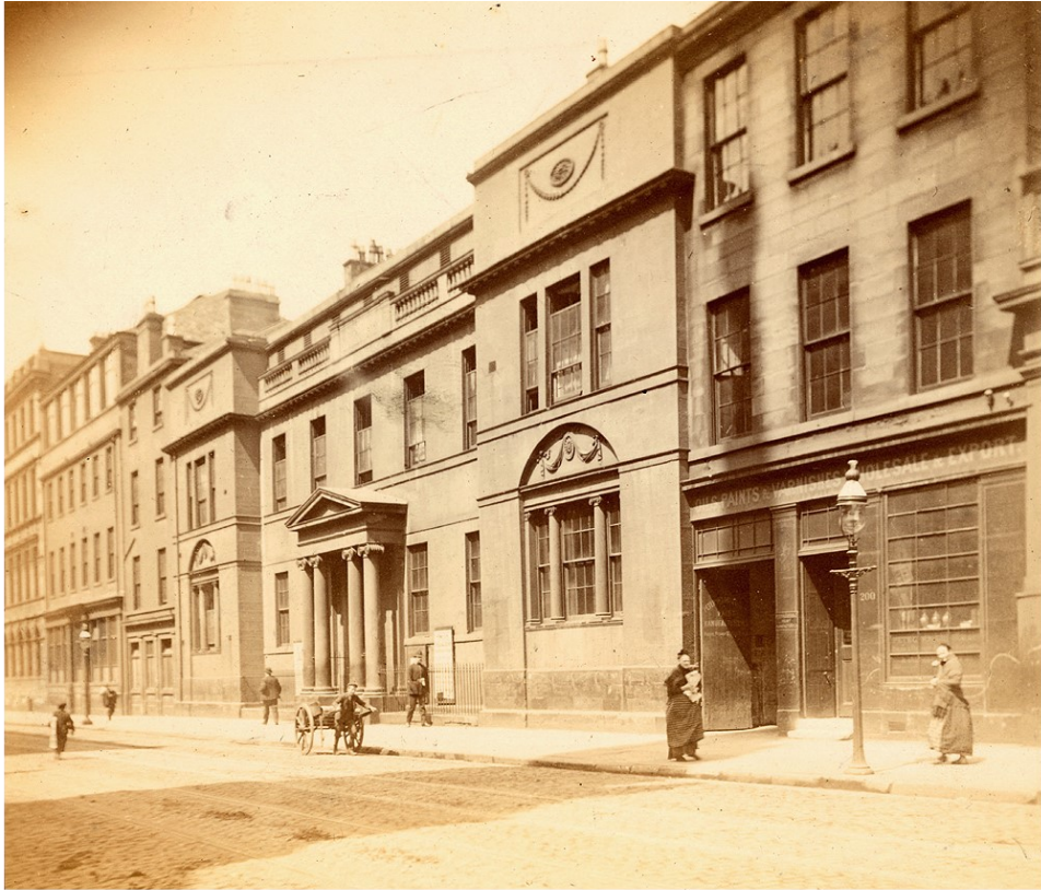
Typical street view
